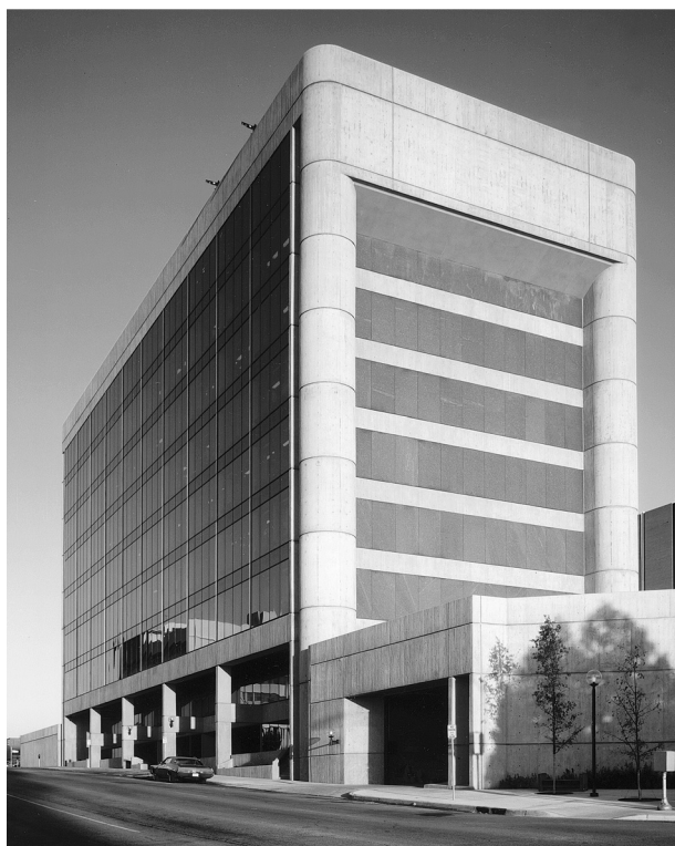
North Façade, Alfred P. Murrah Federal Building
